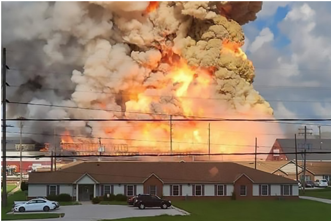
Figure 6 – Battery Recycling Facility Fire in Madison County, IL (2022)
