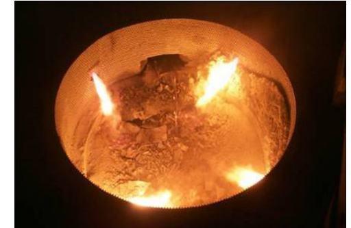
CoJets in Electric Arc Furnace
